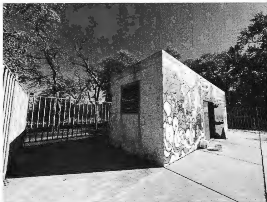
Figure 5 – Pool Filter Building exterior
